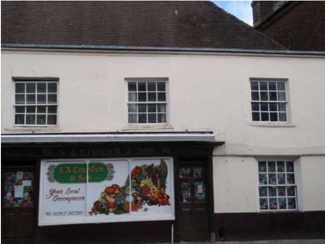
Plate 1. Frontage of building (looking north)
