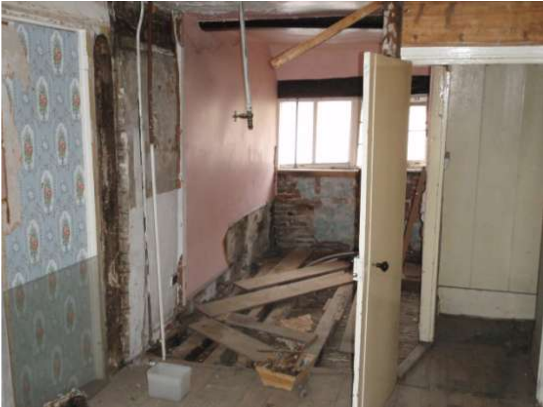
Plate 3. First floor (looking north)
