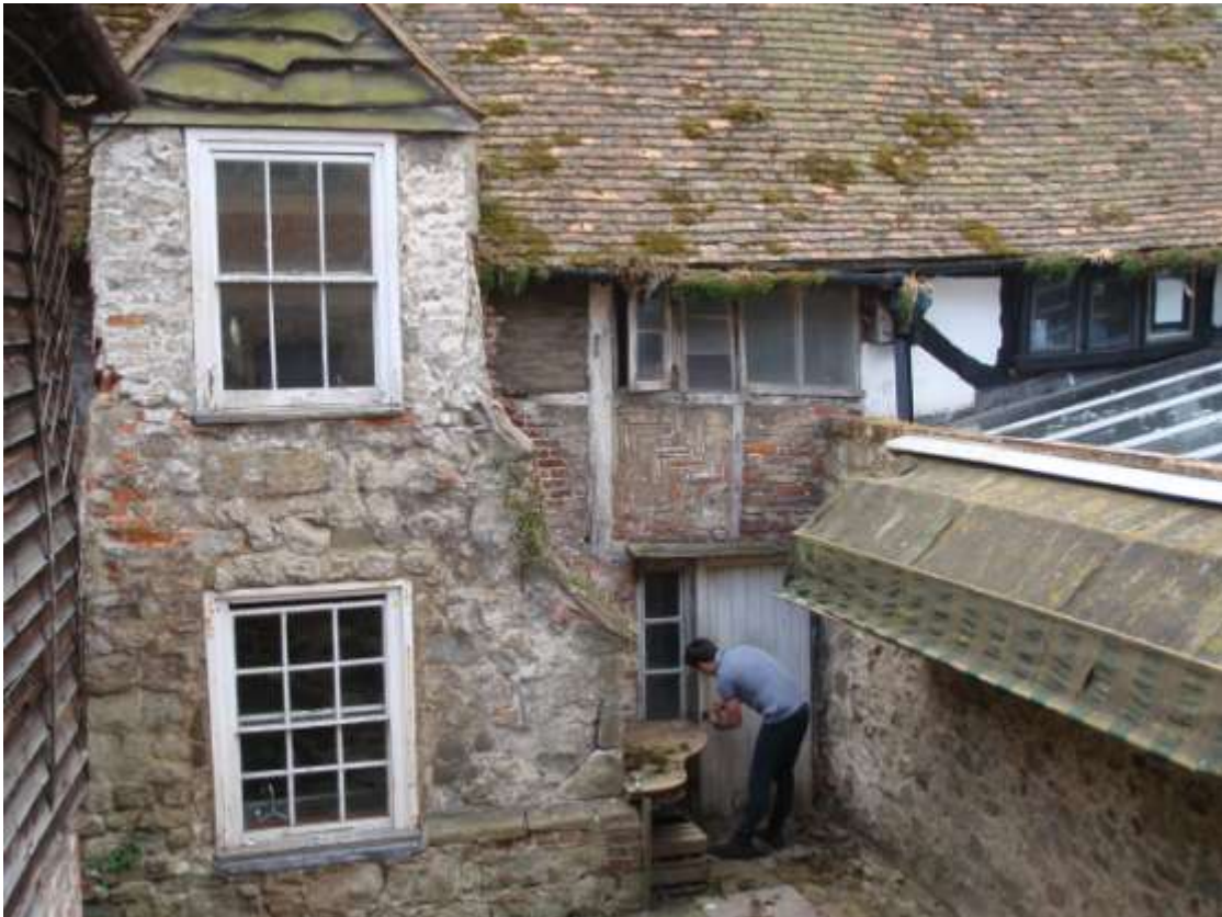
Plate 2. Rear frontage of building (looking south)
