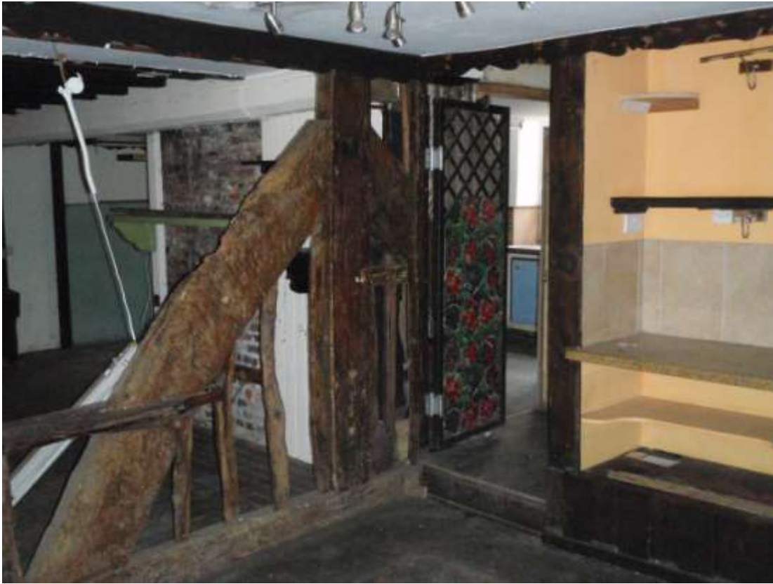
Plate 5. Ground floor-original 14 th century frames and studding
