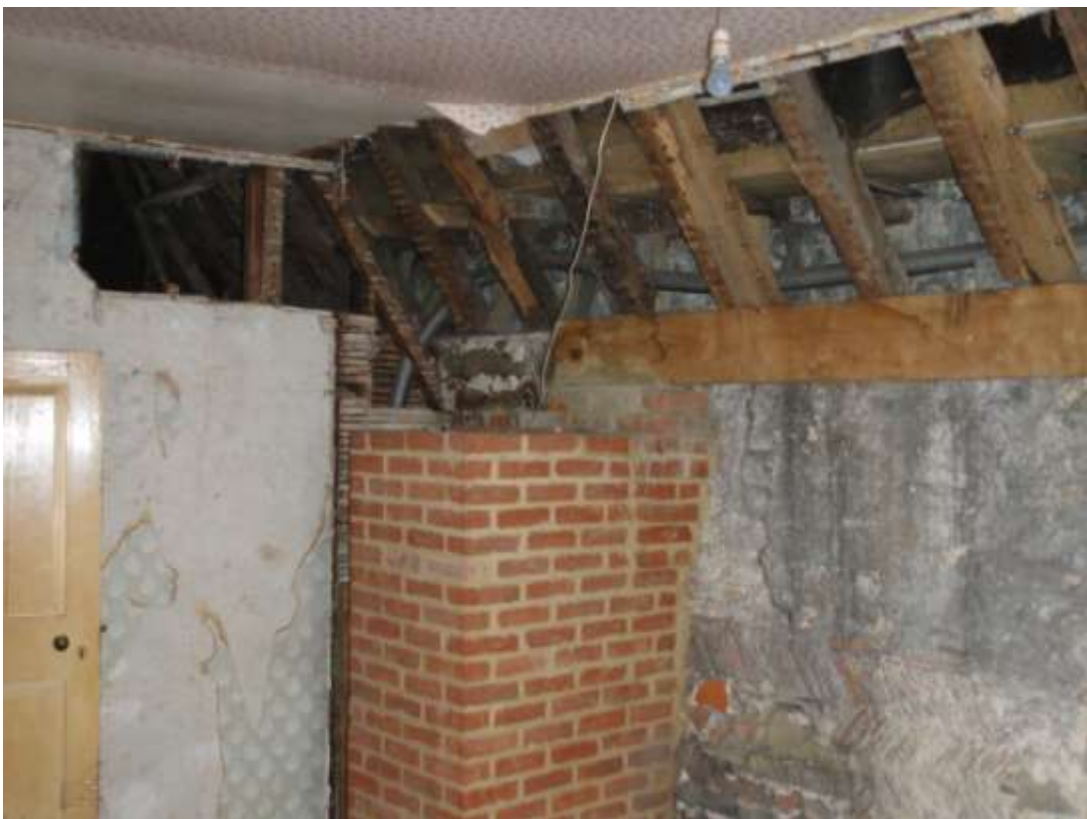
Plate 4. First floor- brick buttress (to be replaced)
